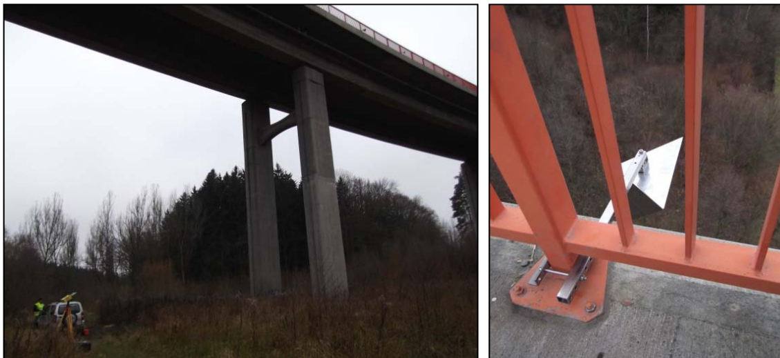
Figure 5 – Measurement situation and corner reflector mounted on the bridge railing
