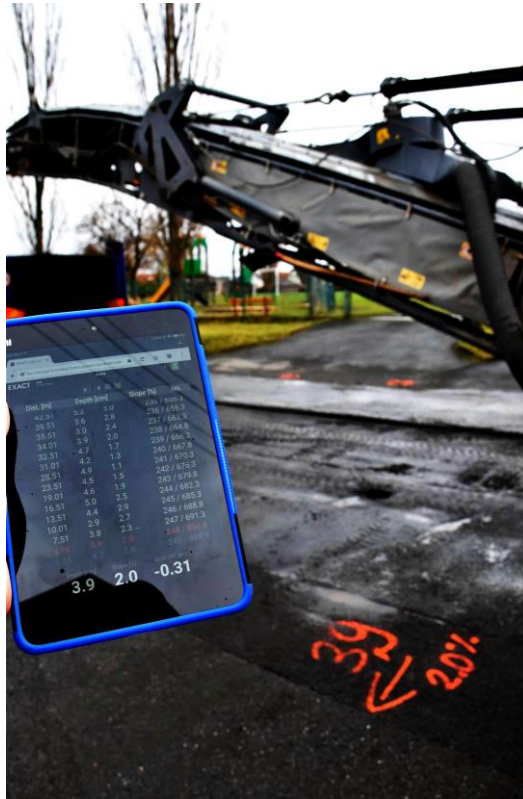
Fig. 5: Exact Street DNA navigation of milling machines using low cost GNSS
