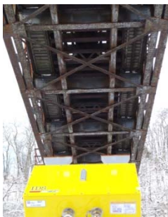
Figure 3 - View of bridge steel crossbeams from the standpoint of the radar.
