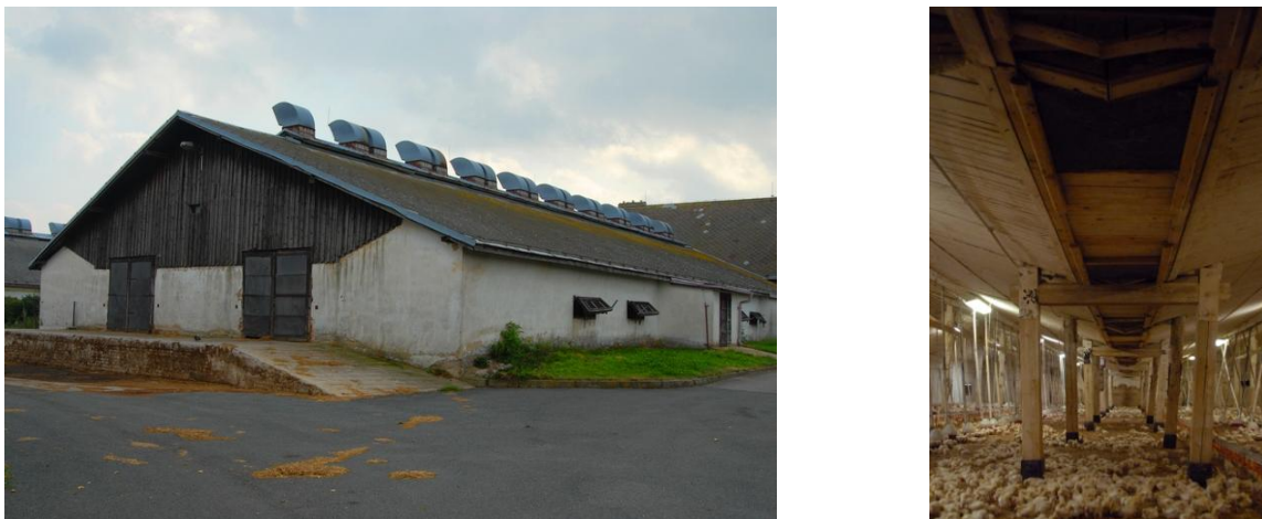
Figure 1. A real, external and internal layout of buildings in University farm. Important are vents in the ceiling of poultry, which are fitted with sliding plates, which are used by operating staff to regulate the intensity (amount) of exhaust air from the broiler house.
